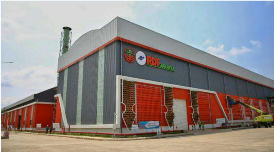
Gambar III.58 Fasilitas Pengolahan Sampah RDF Plant Rorotan
